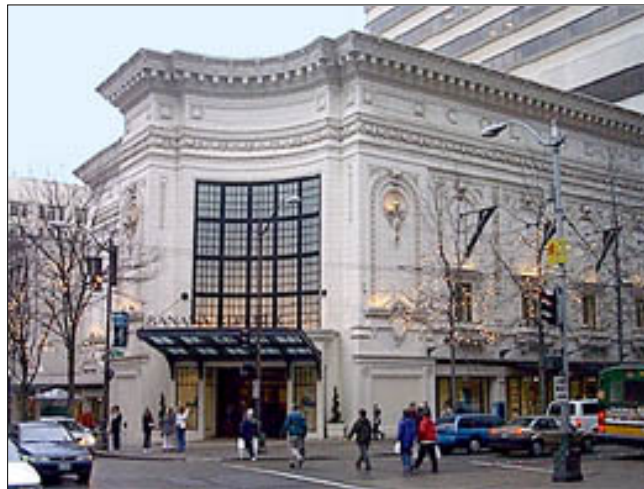
Banana Republic store, former Coliseum (B. Marcus Priteca, 1916), 2001 Photo by Alan Stein
