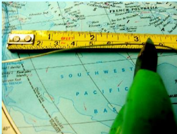
Cut 8 pieces of buss wire. Make each one about 3 inches long just in case!
